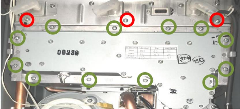
\*Move control board bracket out of way (follow instructions in Section 1).
