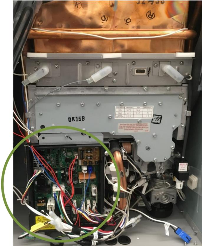
Remove control board Bracket to access water control valves.
