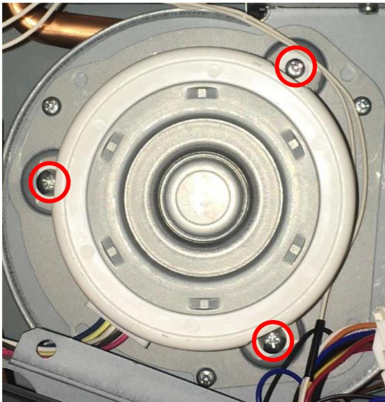
\*Move control board bracket out of way to access blower motor (follow instructions in Section 1).
