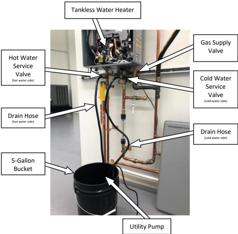
**NOTE:** Flushing instructions utilize a submersible utility pump (provided with the Rheem/Ruud Tankless Flush Kit – RTG20124)
